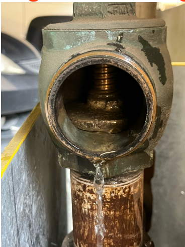
3rd floor East parking garage valve leaking by
