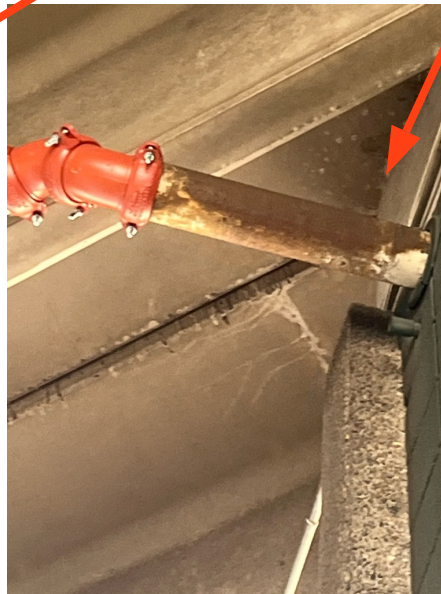
First floor west parking garage leaking at tee
