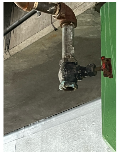
First floor west parking garage 1" valve leaking By
