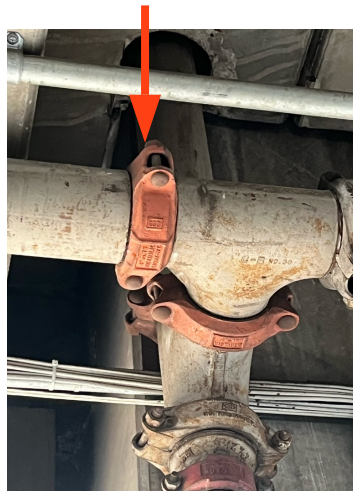
First floor west parking garage leaking at tee
